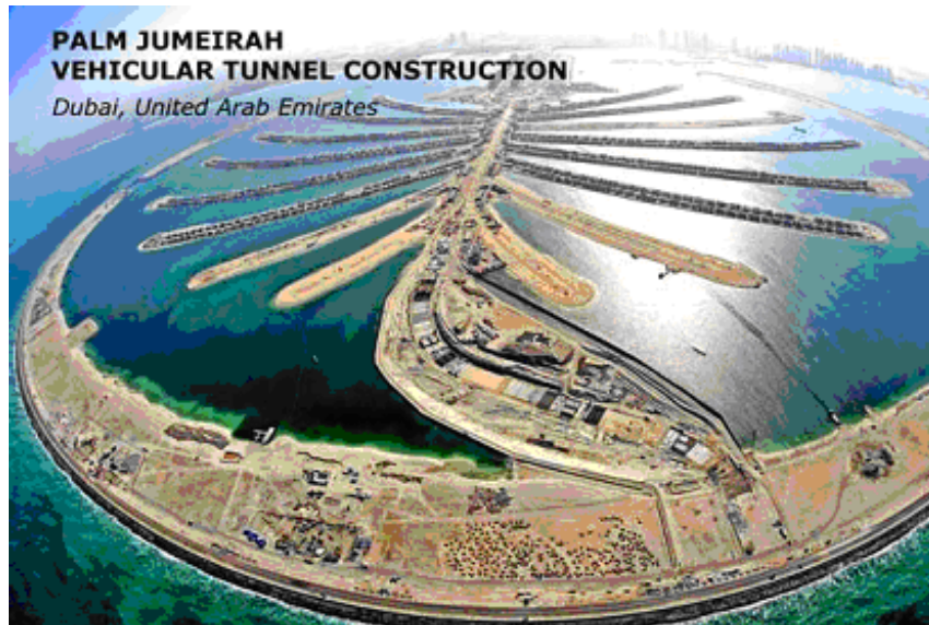
Image courtesy Parsons Corporation
